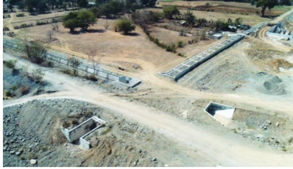
Combined wasteway and cross siphon of ADRIS main canal
