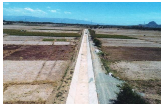
Concrete canal lining along LARIS main canal
