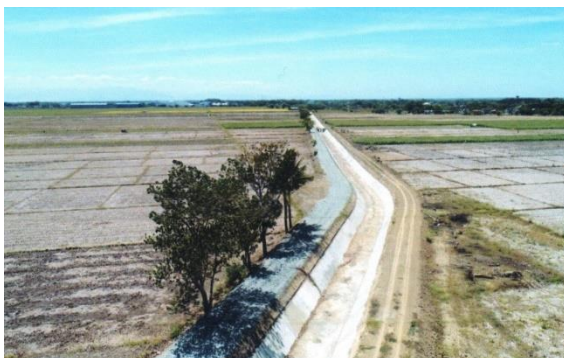
Concrete canal lining along LARIS main canal
