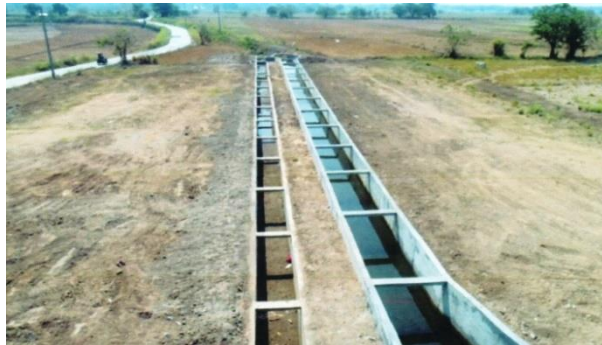
Combined rectangular and supply canal of ADRIS Lateral A
