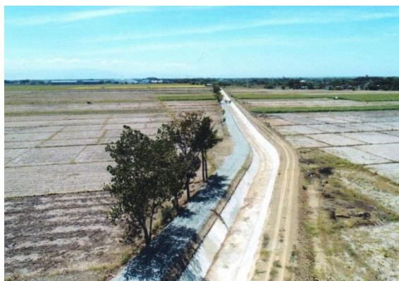
Construction of trapezoidal concrete canal lining along LARIS main canal
