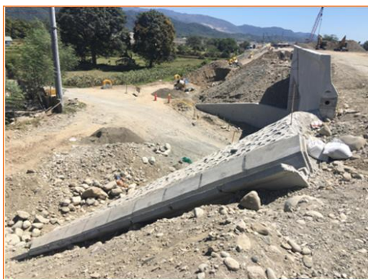
Construction of grouted riprap, North & South bounds – Esperanza Underpass
