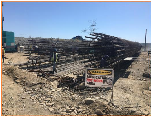
Rebar cage for Bored Pile (100/104) and median barrier Pier 12 to Pier 25- Bued Viaduct
