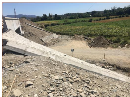
Construction of grouted riprap, North & South bounds – Esperanza Underpass
