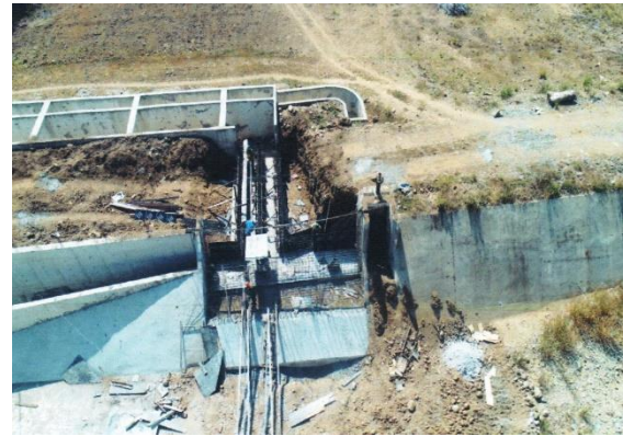
Construction slope protection and headgate of ADRIS main canal
