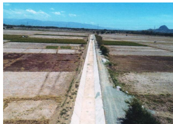
Construction of trapezoidal concrete canal lining along LARIS main canal
