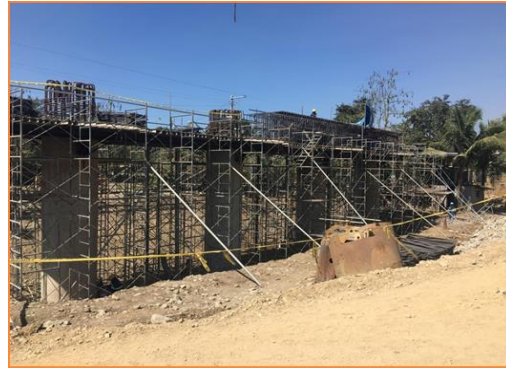
RSB installation at Pier 2 – Provincial Bridge.
