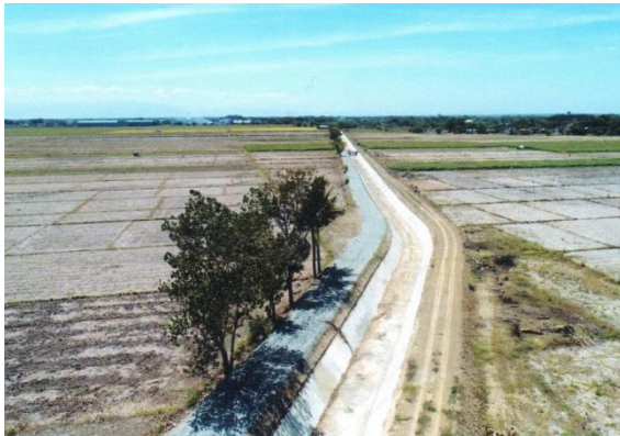
Concrete canal lining along LARIS main canal
