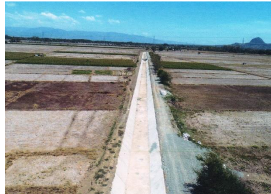
Concrete canal lining along LARIS main canal
