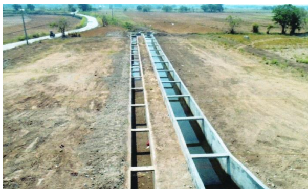
Combined rectangular and supply canal of ADRIS Lateral A
