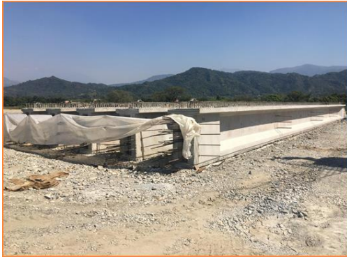
Initial stressing for Sison Interchange.
