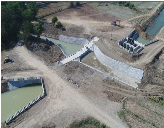
Construction of combined siphon, road crossing & check at ADRIS main canal (left) and construction of ADRIS main canal and appurtenant structures (right) in San Quintin, Pangasinan
