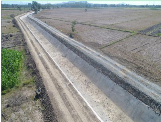
Construction of trapezoidal concrete canal lining & appurtenant structures of LARIS main canal in Rosales, Pangasinan
