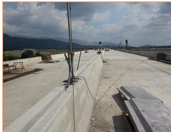
RSB installation for column at abutment B (left) and median barrier Pier 12 to Pier 25 (right) at Bued Viaduct (Binalonan, Pangasinan)
