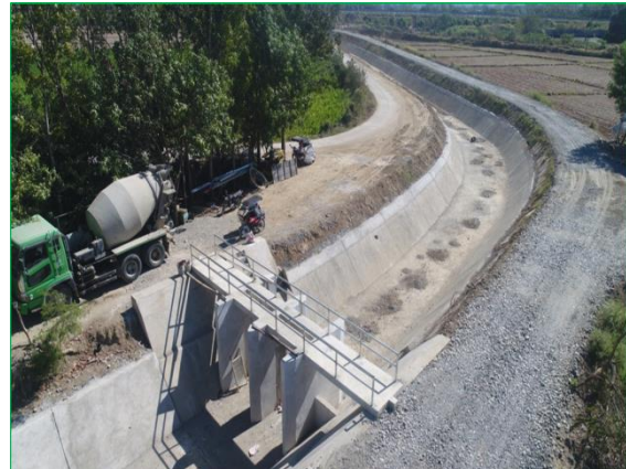
Construction of trapezoidal concrete canal lining & appurtenant structures of LARIS main canal in Rosales, Pangasinan
