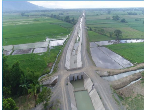
Construction of ADRIS main canal and appurtenant structures in San Nicolas, Pangasinan
