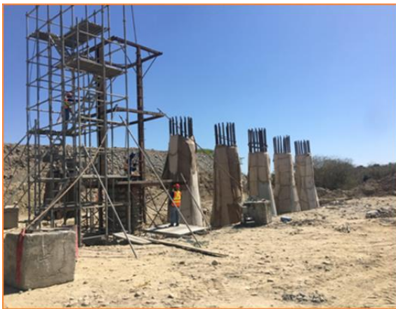
RSB installation for column at abutment B (left) and median barrier Pier 12 to Pier 25 (right) at Bued Viaduct (Binalonan, Pangasinan)
