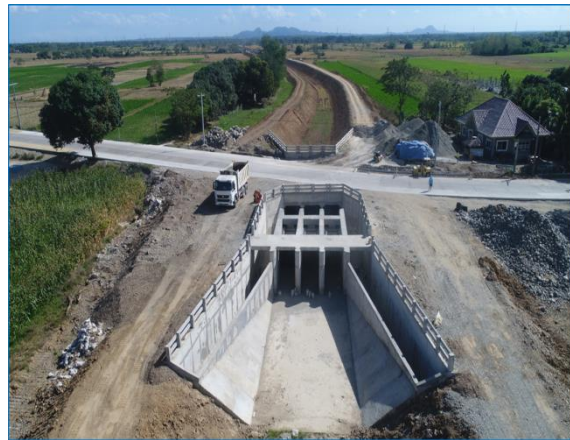
Construction of combined siphon, road crossing & check at ADRIS main canal (left) and construction of ADRIS main canal and appurtenant structures (right) in San Quintin, Pangasinan
