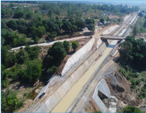
Construction of ADRIS main canal and appurtenant structures in San Nicolas, Pangasinan
