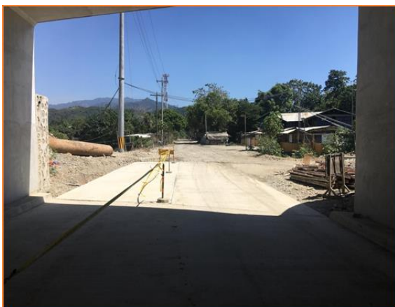
PCCP completed at North and South bound Udiao 1 Underpass (Rosario, La Union)
