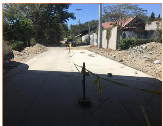
PCCP completed at North and South bound Udiao 1 Underpass (Rosario, La Union)
