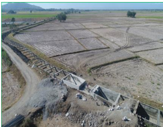
Construction of thresher crossing (left) and rectangular concrete canal lining (right) of LARIS lateral A in Rosales, Pangasinan
