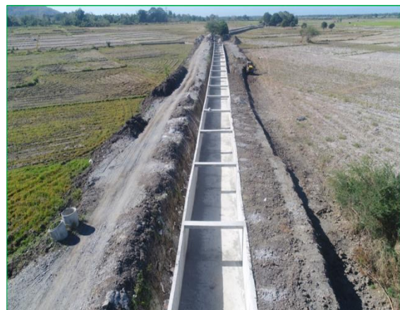
Construction of thresher crossing (left) and rectangular concrete canal lining (right) of LARIS lateral A in Rosales, Pangasinan
